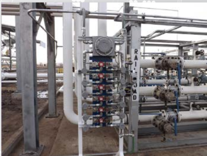
Additive Injector Install– Hammond, Indiana
